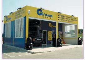
Innovative concept of workshops / boxes of 60 m² that delimits a workshop, an oil change zone, an office and a warehouse with equipment for the lubricant extraction and supply.
